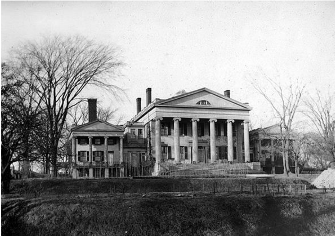
Parker House in New Bedford, Mass. 1834.
