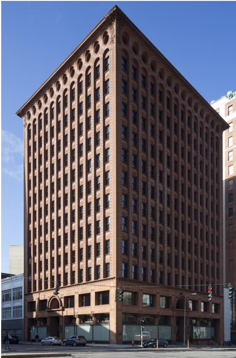
The Guaranty Building (now the Prudential Building) Buffalo, New York, 1895, Adler and Sullivan
