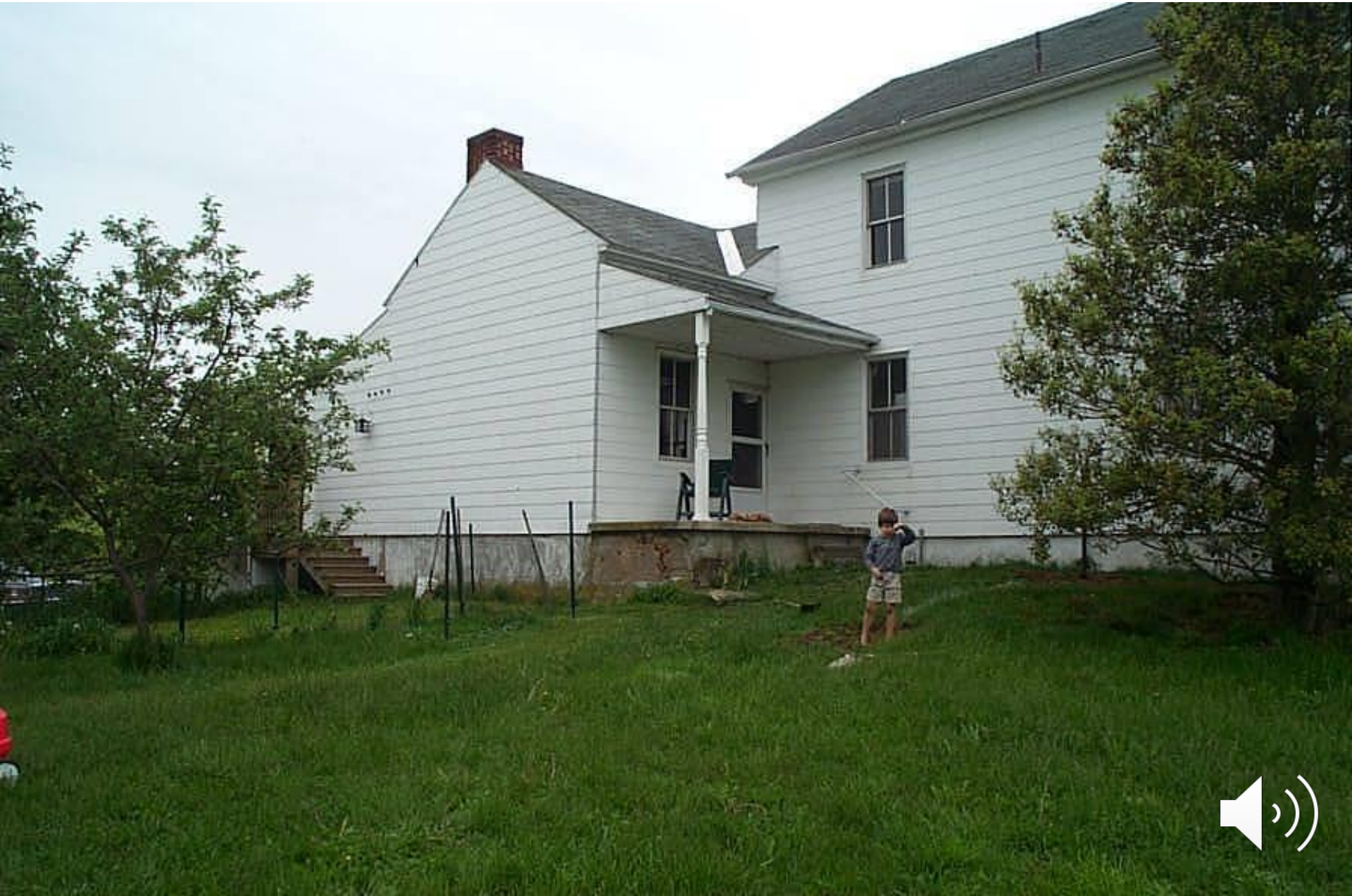
1877 Wunderlich Pennsylvania farmhouse and barn (Post & Beam, Mortise & Tenon construction)
