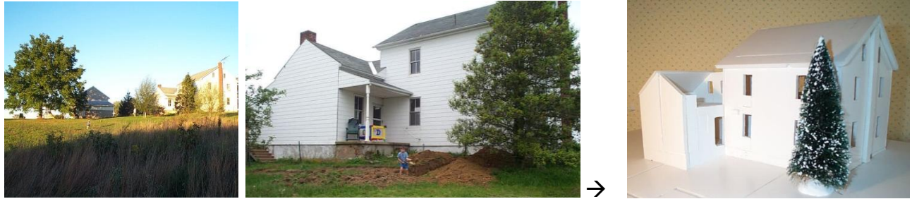
Figure 3. Structure before new architecture ( digging started in Photo #2 ), and foam-board model (2000).
