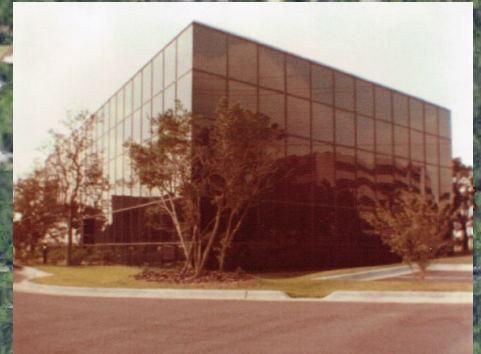
Recent CURTAIN WALL
