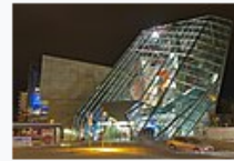
UFA-Palast in Dresden, Dresden, Germany, by Coop Himmelb(l)au
