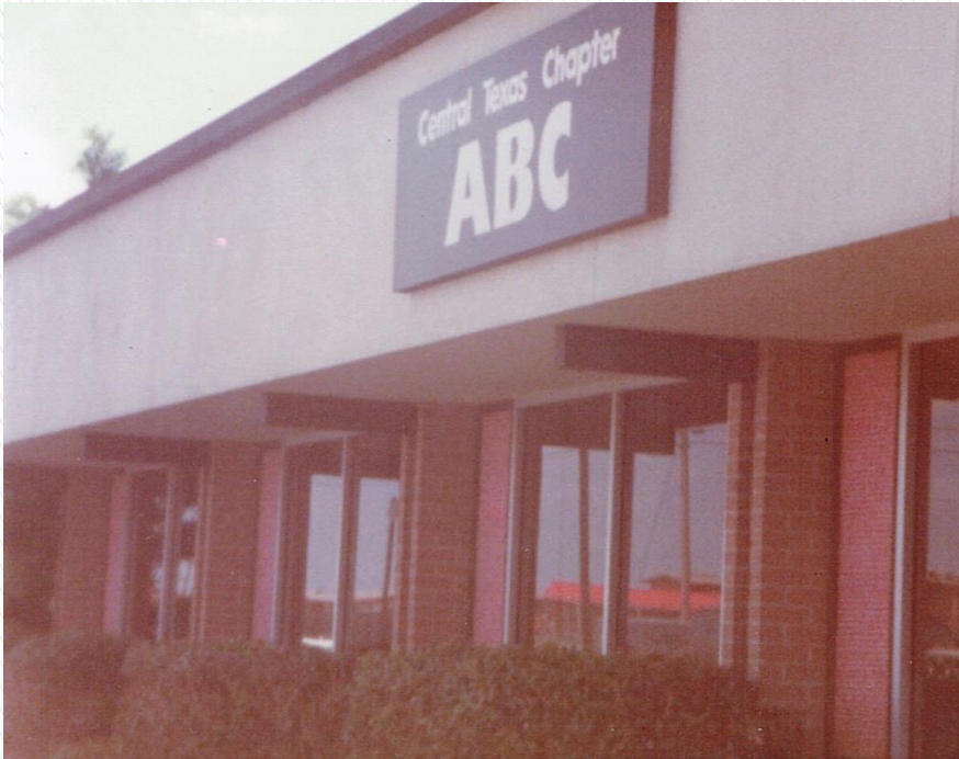
Worked in "ABC" Plan Room used by all contractors in Austin
