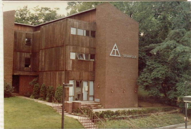
DESIGN-BUILD OF FRONTAGE LANDSCAPING AND RETAINING WALL
